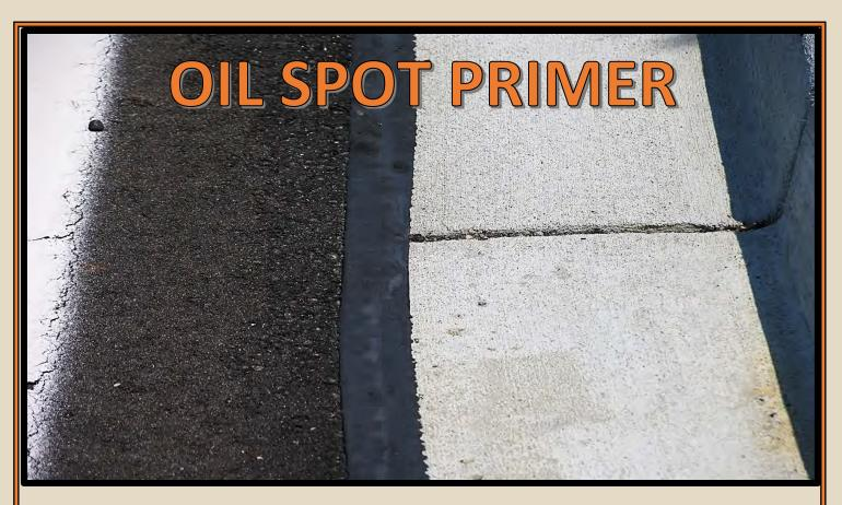
Brewer Cote Oil Spot Primer is a modified latex acrylic that has been formulated To help Pavement Sealers adhere to existing stained surfaces. Added ingredients improve the penetrating ability of our primer and thus gives added future protection. For use on all Parking Lots, Aprons and Driveways of asphalt construction.
