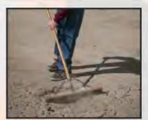
To begin, use a wire brush and compressor to sweep and blow the dirt out of the hole.
