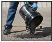
Flow material into damaged area to just-blow grade.
