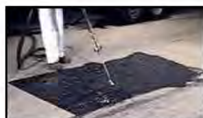
Flood with Concrete Welder.
